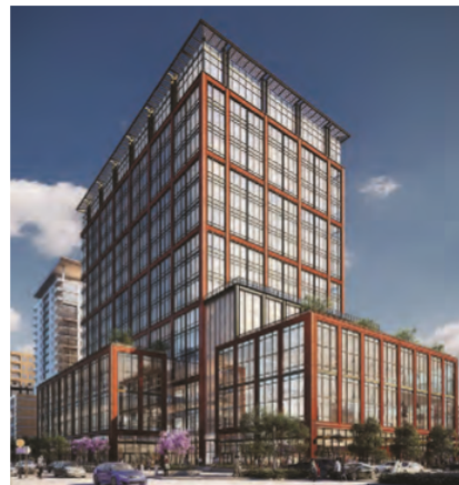
Related Cos' 360 Rosemary office tower under construction in downtown West Palm Beach.
